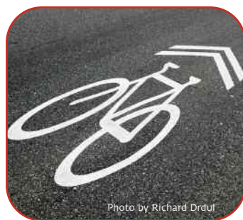
Where a street isn't wide enough for dedicated bike lanes, pavement markings sometimes nicknamed "sharrows" formally indicate a bike route and shared-use lane.
